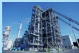
Bucket elevator for biomass power plants (2016)
